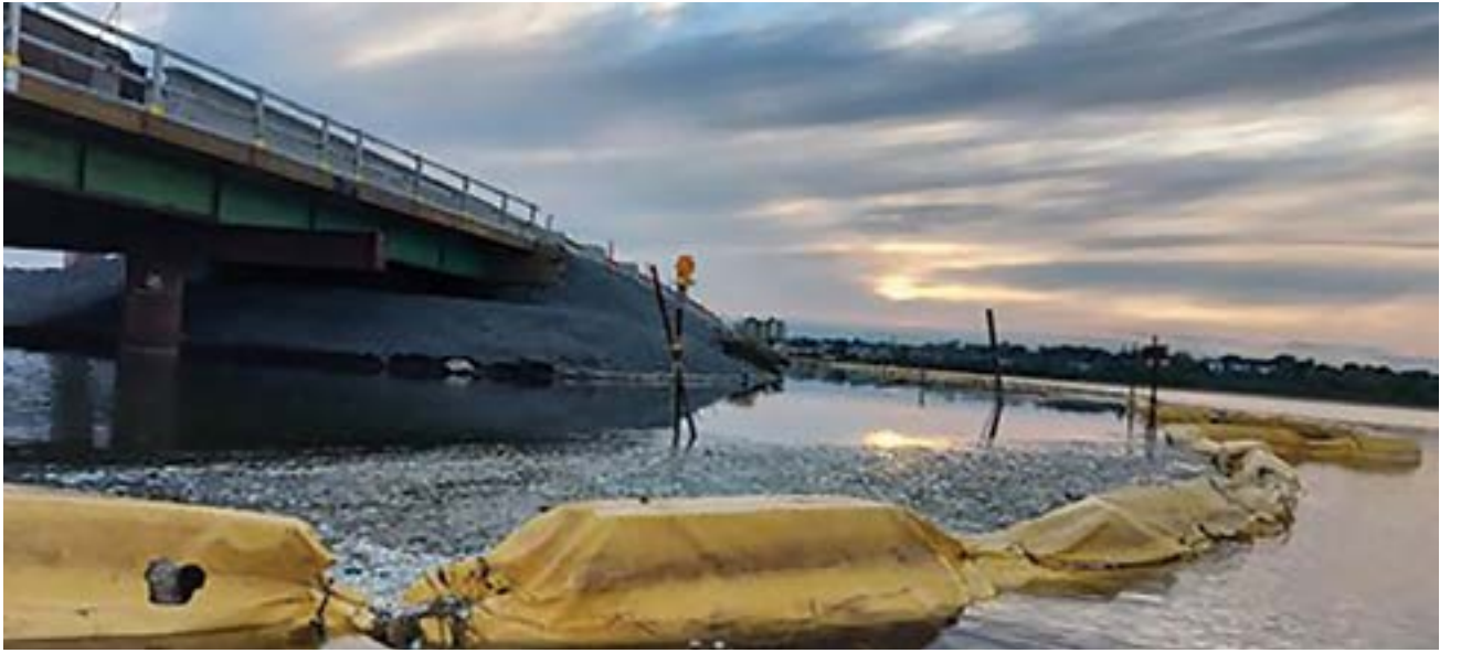
Styrofoam gathers at the base of the under-construction Third Crossing. PHOTO CREDIT: Carl Hanna
